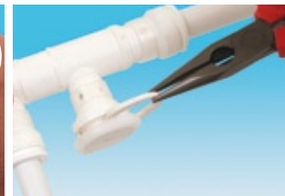
Reusing the connection: remove the clip from the stopper using pointed pliers.
