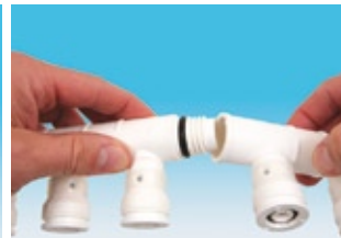
Screw the extension onto the manifold.
