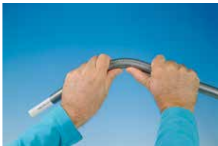
Bending with an external bending spring
