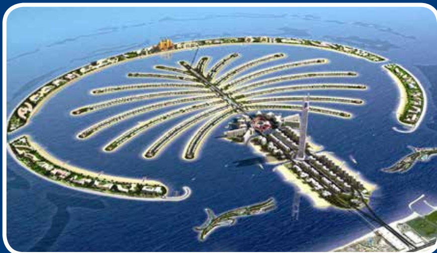
Henco provided all the gas pipes and fittings for Palm Jumeirah (Dubai)
