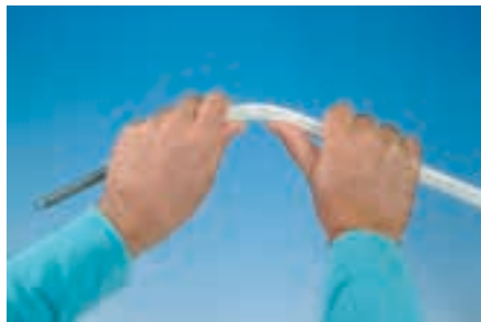
Bending with an internal bending spring
